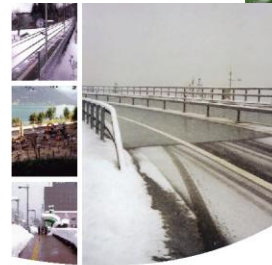
GEOHERMAL SNOW MELTING AND DE-ICING
