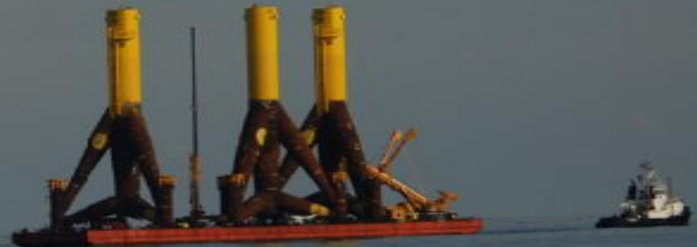
Tripod foundation (760 tons)
