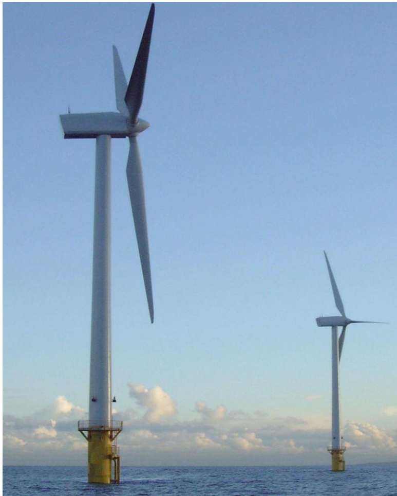
E.ON Offshore Wind Farm Blyth, UK, 4 MW
