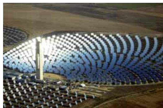
Source: ESTELA (central receiver technology)
